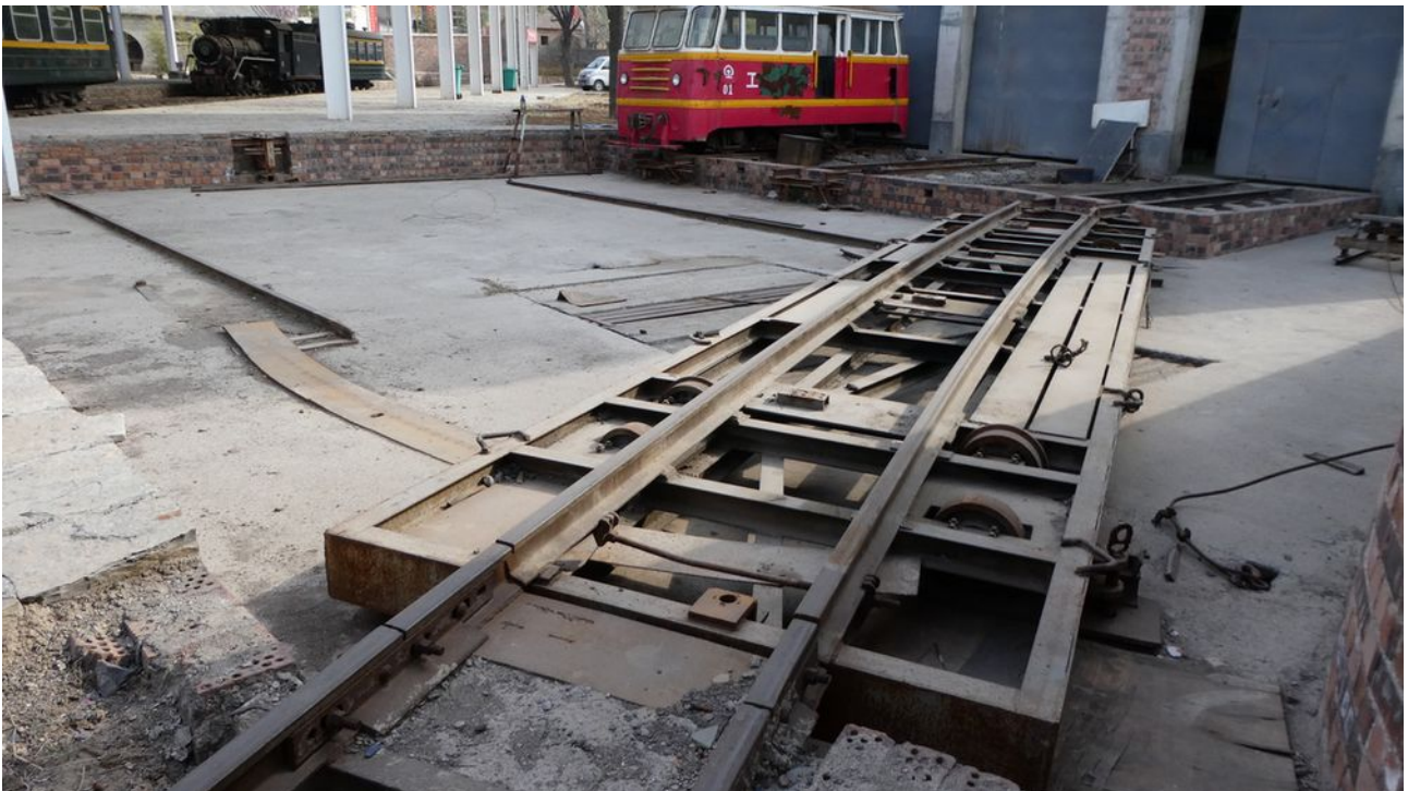
The over-engineered swivelling traverser at the depot. In order to enter the depot, the loco must be positioned on the traverser, the traverser swung left and then to access the second and third roads, the traverser needs to slide sideways. Both rollers and wheels with flanges are needed as well as a cable to pull the traverser from either side. A simpler solution would have been to build
