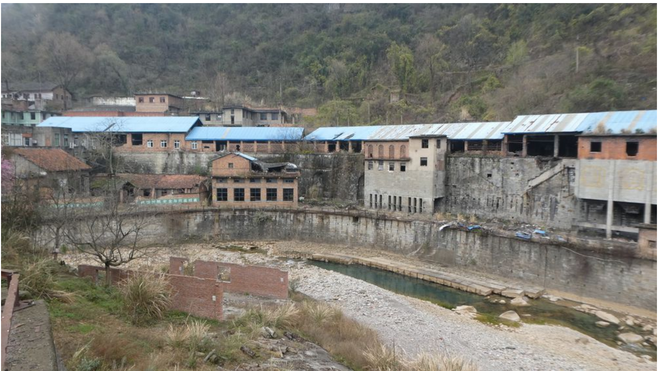
The mine at Yujiabian. In 2014, the mine was being salvaged prior to sealing up.
