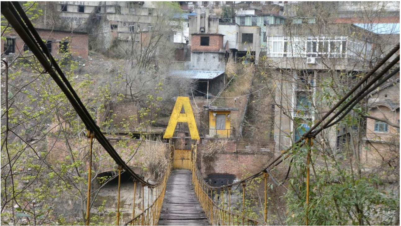
The bridge to the mine with a locked gate under the A. (What does the A stand for?)
