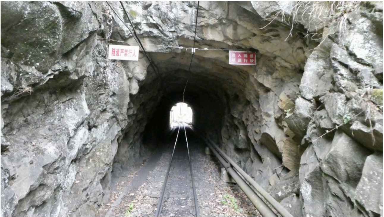
Tunnel No. 2 is a rock cut tunnel
