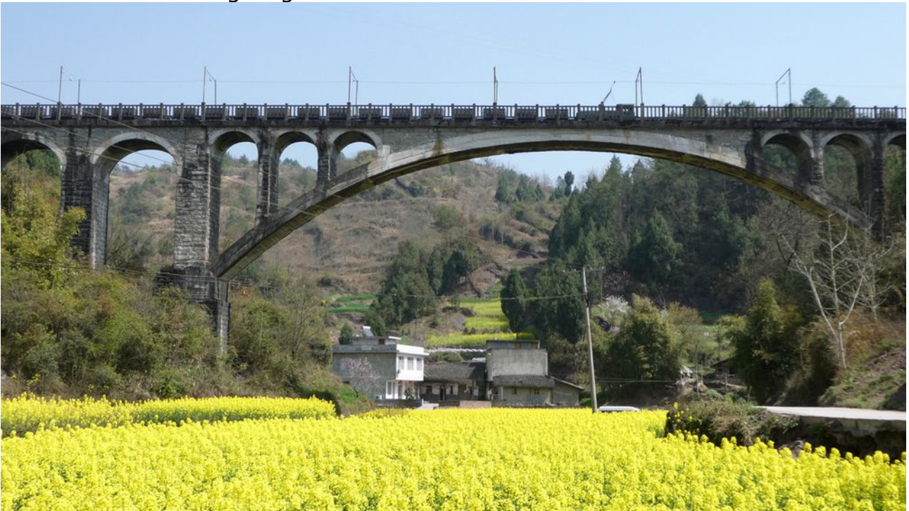
Another line, another big bridge. The empty coal train is visible but mainly behind the bridge railings.
