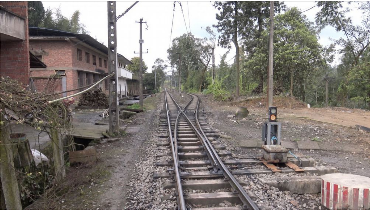
Full trains use the through line and empties go into the loop. This shot is looking towards Honglu.
