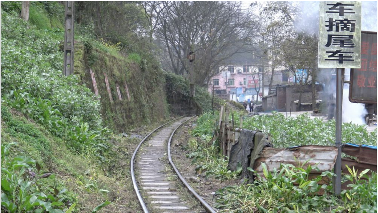
Looking the other way, this is truly the end of the line around Km 23.
