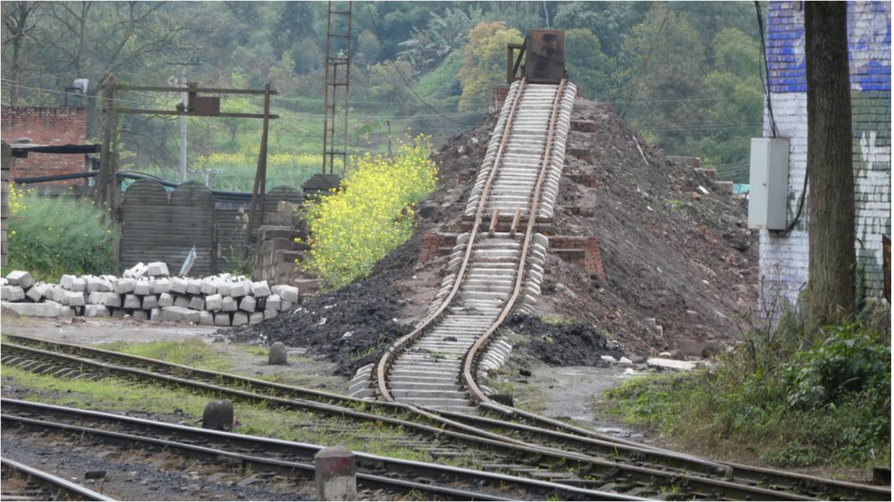
A newly constructed runaway ramp at Honglu. It may replace a previous version. The trains have only loco braking so this may be needed at times.
