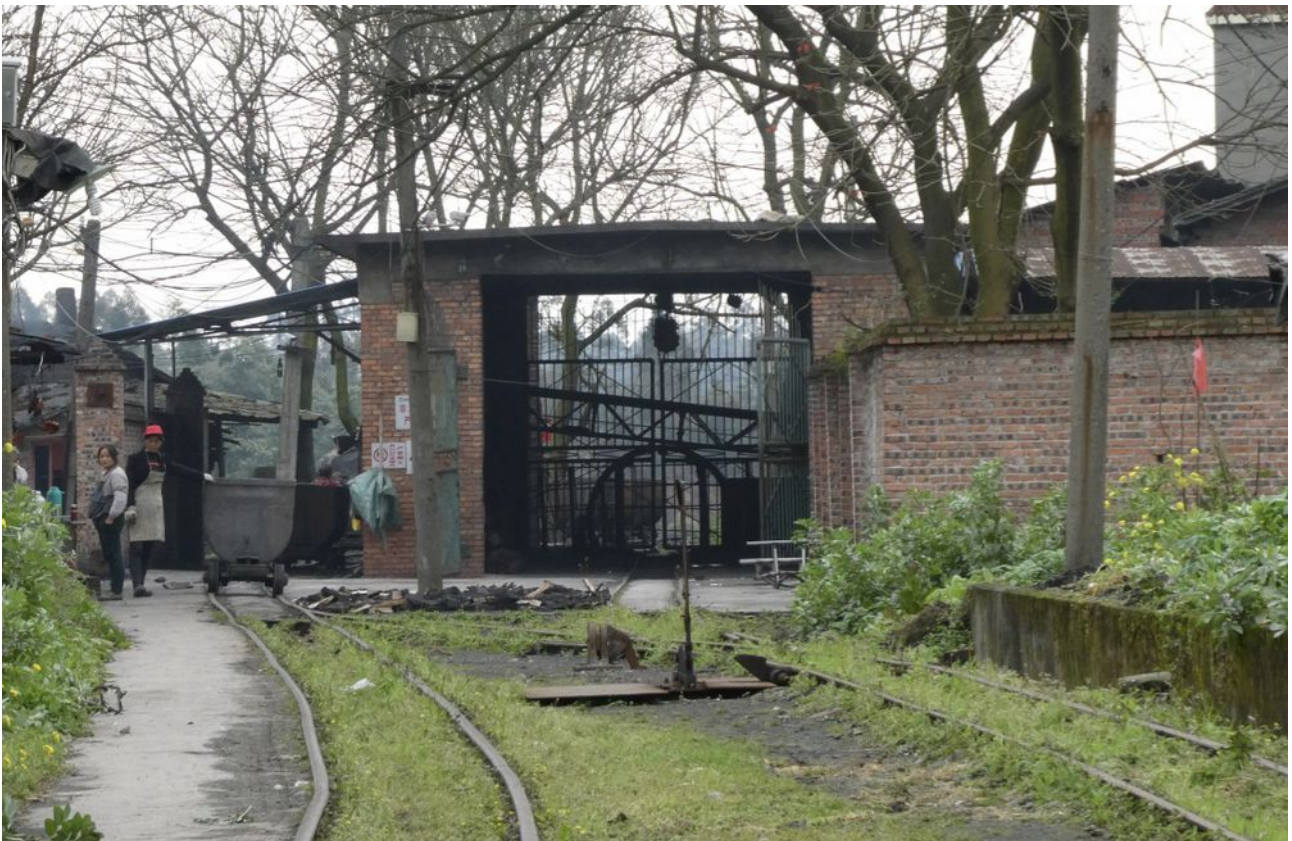
On a higher level there is a 600mm line formerly with overhead wires but now using a battery electric loco. The line runs for around 500m from the tippler shown to a works yard. Its purpose is not known but it is reported in daily use.
