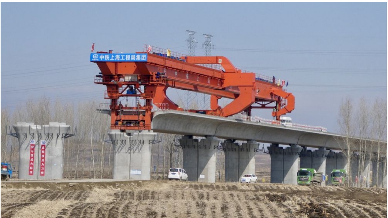
Equipment for moving the spans for the high speed train into place.
