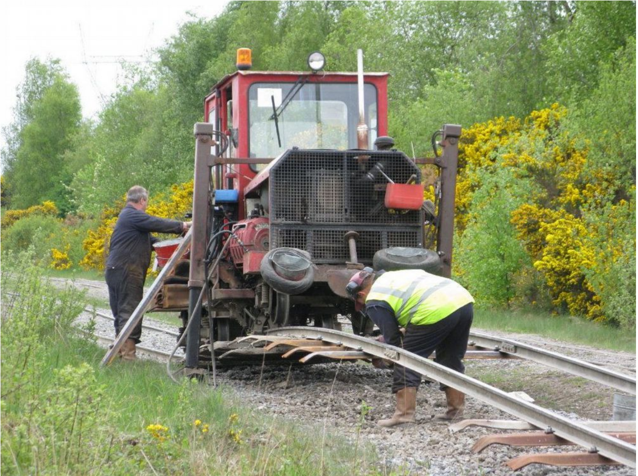
Track repair near Shannonbridge, Ireland
