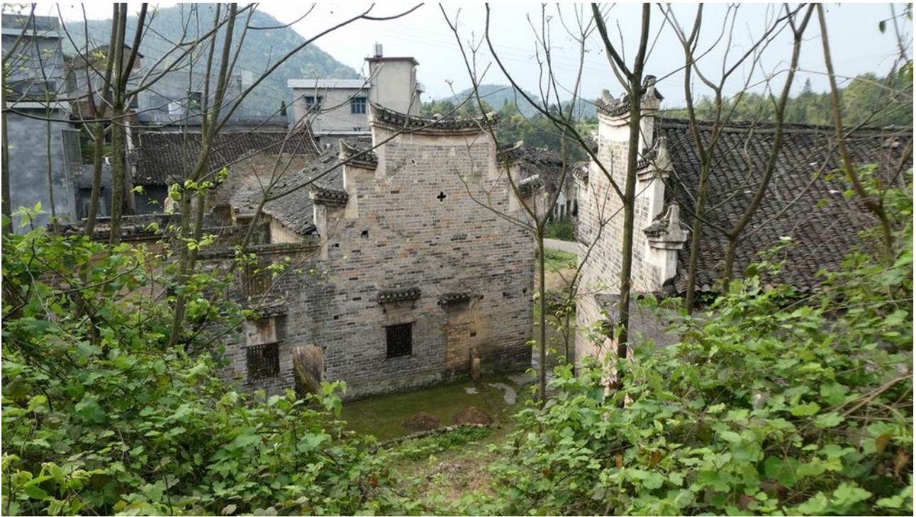
Old houses mainly abandoned.
