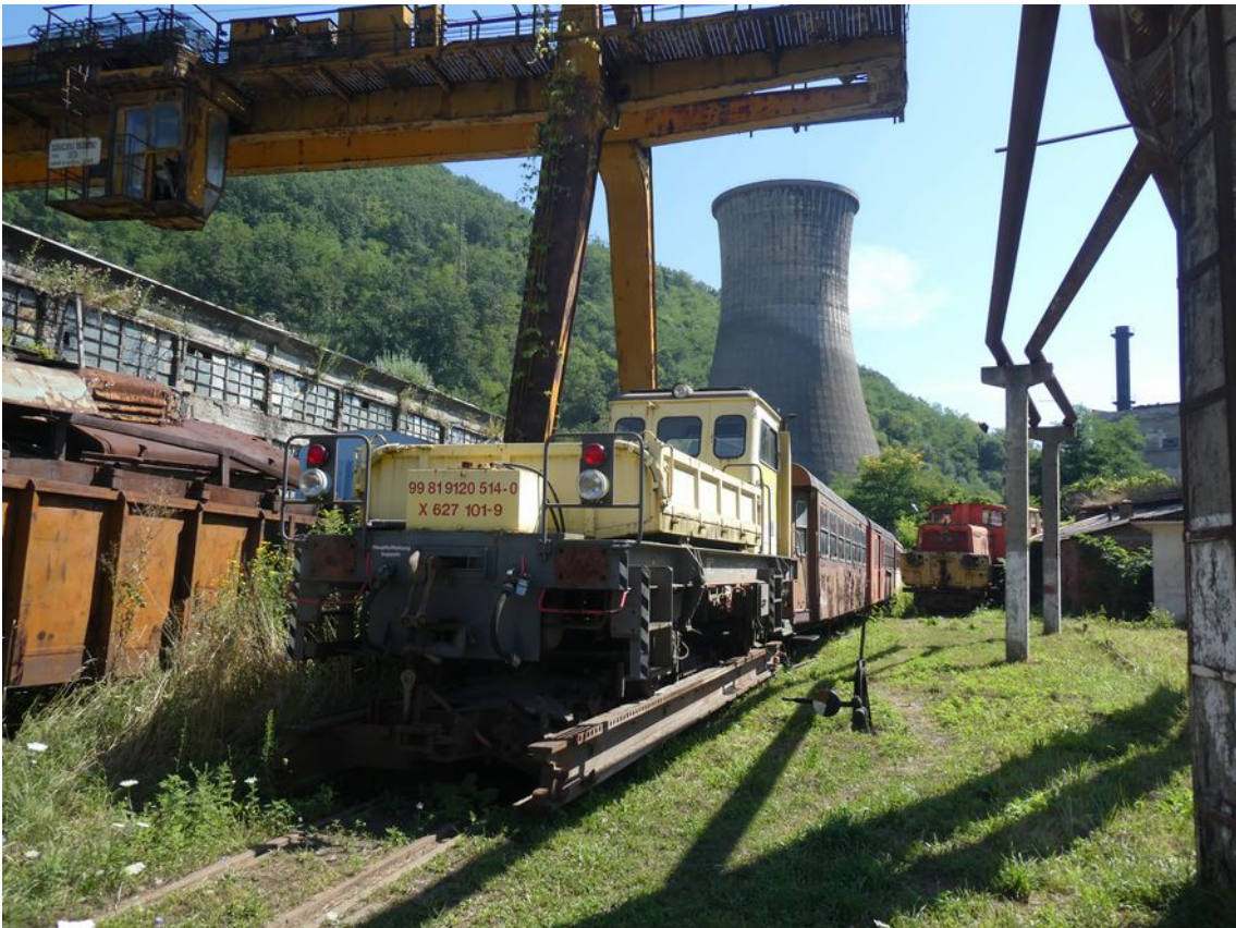
In the shadow of the cooling tower for the town central heating plant, among other things a standard gauge track vehicle on a narrow gauge transporter wagon.
