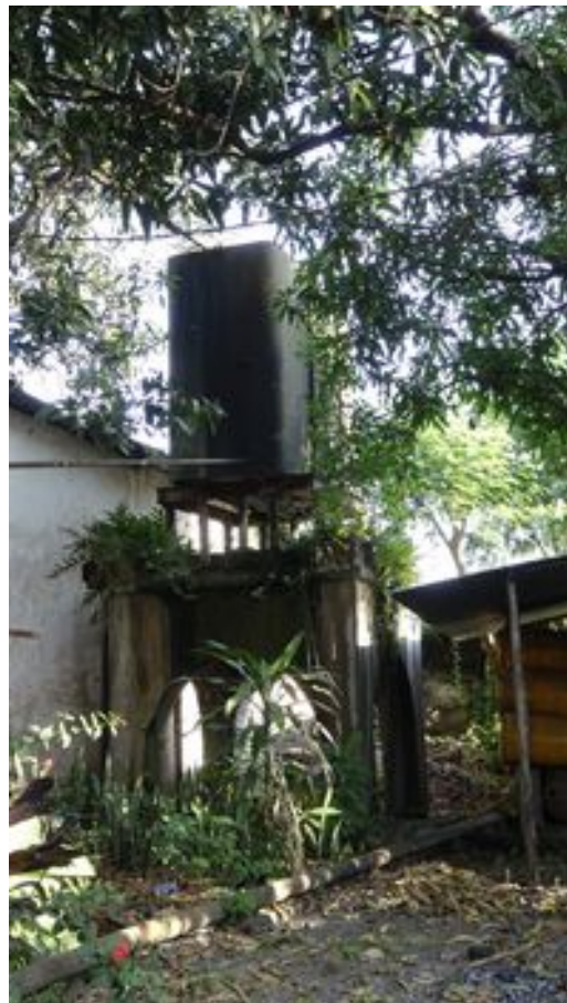
Water tank beside the roundhouse likely to date back to the steam era.
