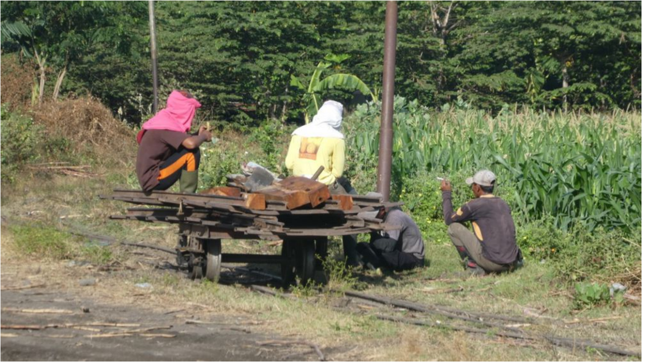
The track crew waiting to go out attached to the rear of a train of empties with two sets of points and some sleepers loaded on a flat wagon.
