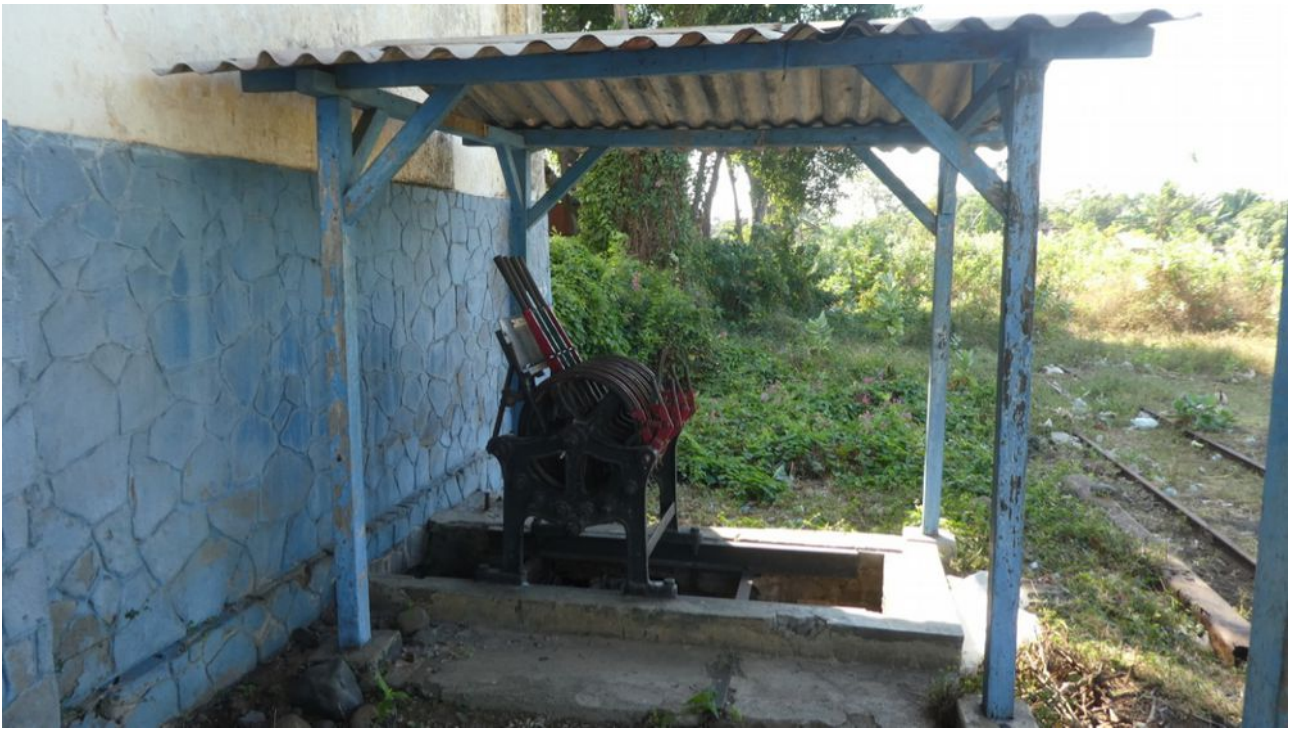
The signal and possibly point controls at the east end of the station platform. The levers are labelled Dari (from) Panarukan and Dari (from) Prajakan.
