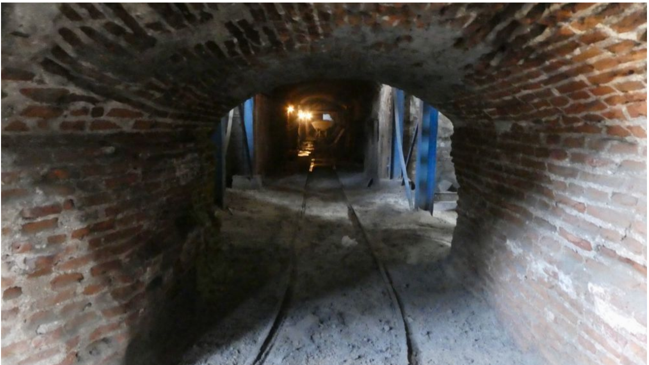
This tunnel goes under the boilers to remove ash in V-skips which will be pushed out by hand. Try to imagine the heat in there!
